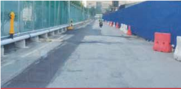
3. The speed bump on the road is not visible on the road
