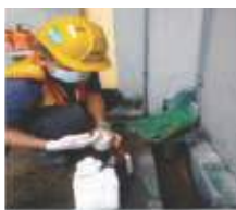
Location Plant room
