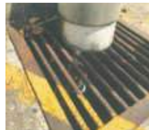
Location Gate 2 (Additional Point)
