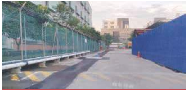
6. The wall metal cladding construction is not visible at night
